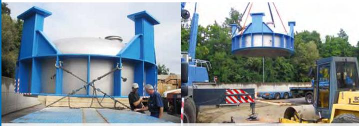
Loading of the timber processing units in Germany which weigh 35 tonne
