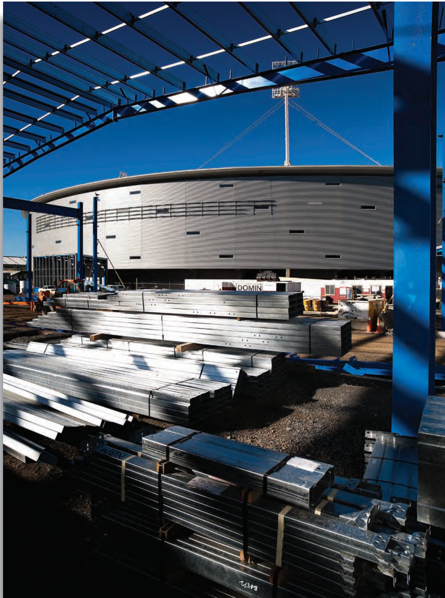
Mainfreight's new facility in Wellington is taking shape
